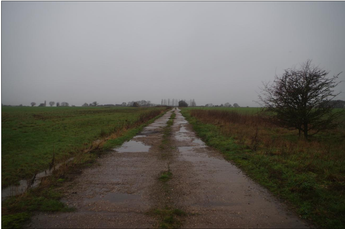
Plate 2) View of what remains of the former northwest-southeast aligned runway, facing northwest
