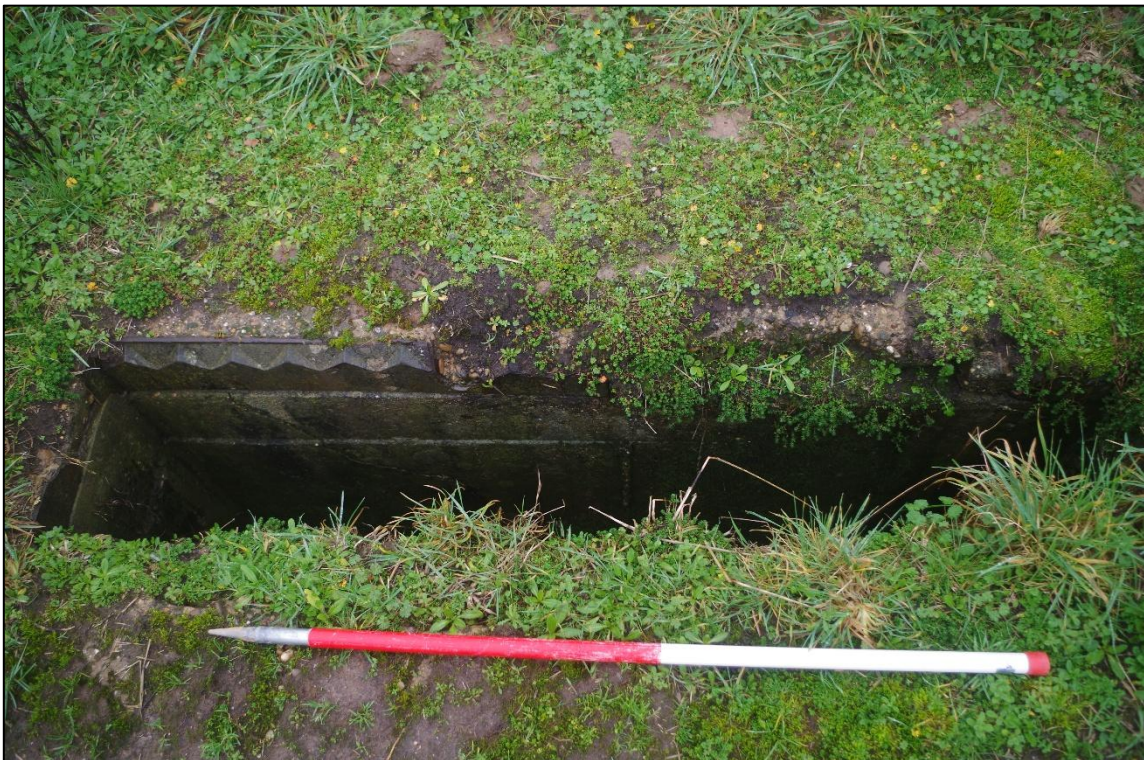
Plate 3) exposed section of the former northwest-southeast runway drainage, facing northeast
